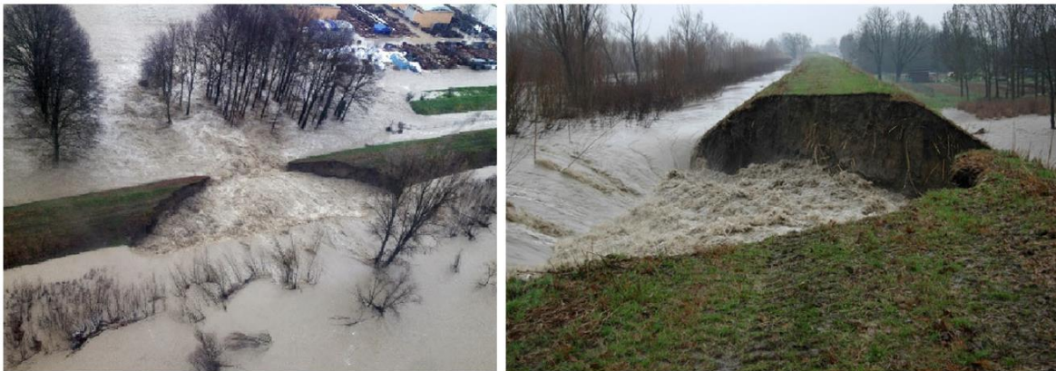
Figure 1: The levee breach on the Secchia river at the end of the evolution
